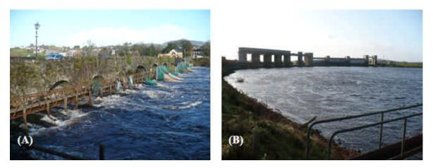
Figure 7-2: The Killaloe eel weir (A) and the Parteen regulating weir (B) on the lower River Shannon.
