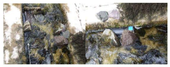
Figure 3-4: Pipe traps set in the fish pass at Galway weir on the Corrib
