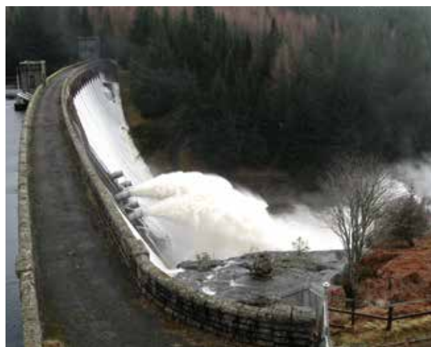
Figure 3.8 Laggan Dam, Highland, Scotland. By altering the pattern of natural flows and sediment movement, dams and associated flow regulation can affect habitat downstream (© James Hutton Institute).
