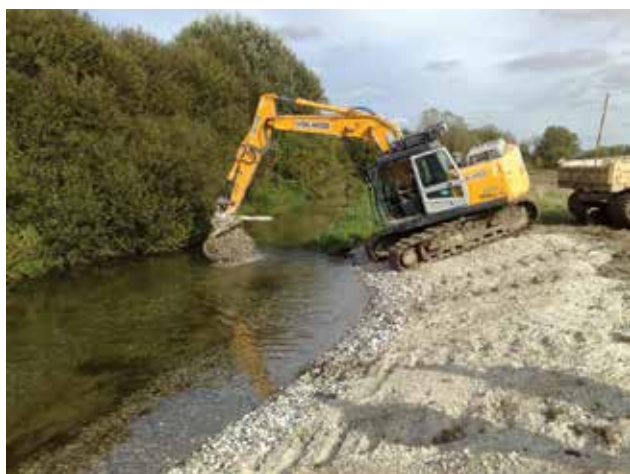
Figure 5.6 (Left) Adding locally sourced gravel to the River Wylfe in Wiltshire. This can restore river-bed levels, floodplain connectivity and flow velocities for spawning fish, macroinvertebrates and plant communities (© Hampshire Aquatic Services). (Right) The Ben Gill and River Ehen in Cumbria. The Ben Gill was reconnected to the River Ehen in 2014 to restore natural flows and sediment supply (© Baptiste Mareau, Northern Rivers Institute).
