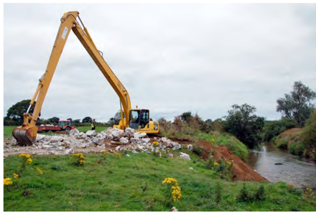
Plate 11 and Plate 11.1 Constructed of rubble mat on Mulkear River (August, 2012)
