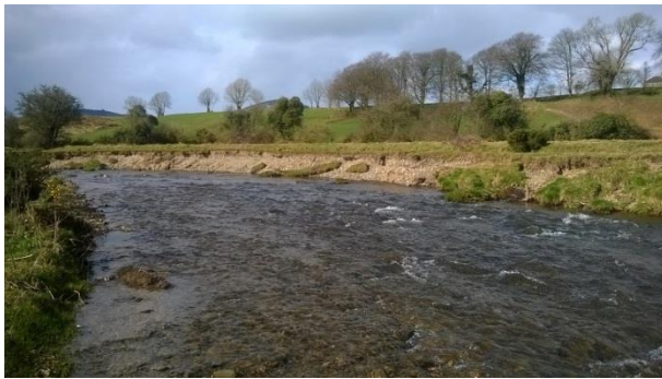
Bank protection (80m) with V-notch weir and scour-pool also random boulders (8) and grade river on Lhs. Cattle Drinker (Site 7.)
