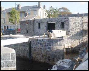
Figure 36. Weir refurbishment works in progress
