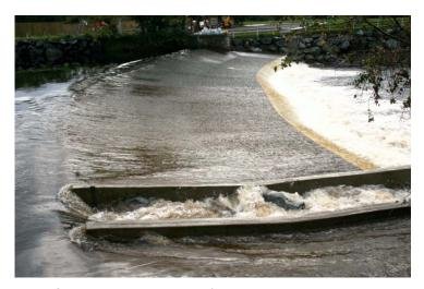
Figure 11. Temporary Solution: A ramp type fish pass was installed as an interim measure
