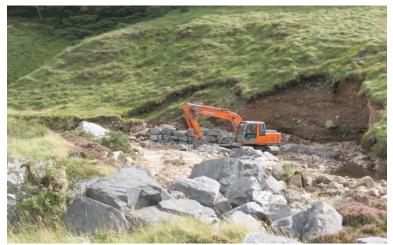
Figure 4. Installation of rock armour on Lowerymore River to prevent erosion
