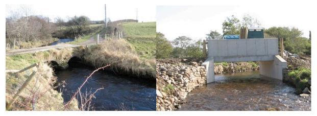
Figure 16. Bridge over Abbey River (for replacement). Abbey River Bridge completed works.
