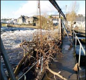
Figure 35. Pre works – corroded and unsafe superstructure with debris build up on the upstream face of the weir
