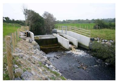
Figure 14. Small scale hydropower facility on Ballintra River, Cavan, showing fish passage facilities
