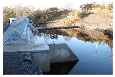
Figure 13. Lowerymore River – completion of modified hydropower intake and improved fish pass
