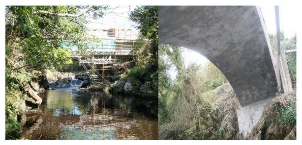
Figure 17. Westbrook Bridge on the Crana River during restoration and Westbrook Bridge with the under-span works completed
