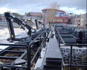
Figure 37. Refurbished weir with new hydraulically operated gates in open position. Cranes for debris removal and heavy lifting also visible.
