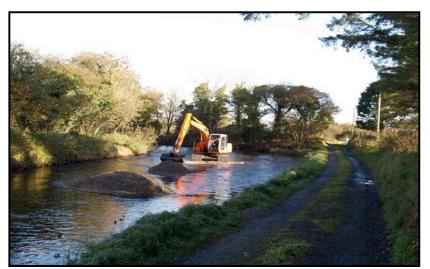
Figure 9. Spawning gravel being introduced and spread in the Cloonaghmore River (Palmerstown, Mayo)
