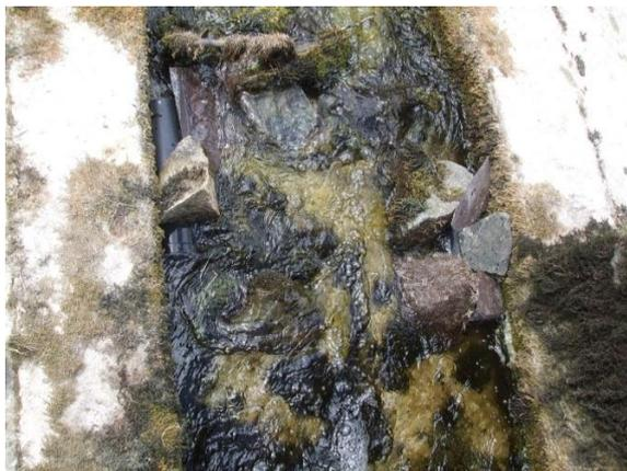
**Plate 4-2 Elver pipe traps set in the fish pass at Galway weir**
