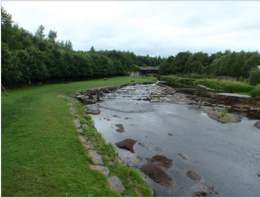
Plate 2.4. A weir on the River Nore at Castletown, Co. Laois, modified by installation of a rock-ramp fish pass.
