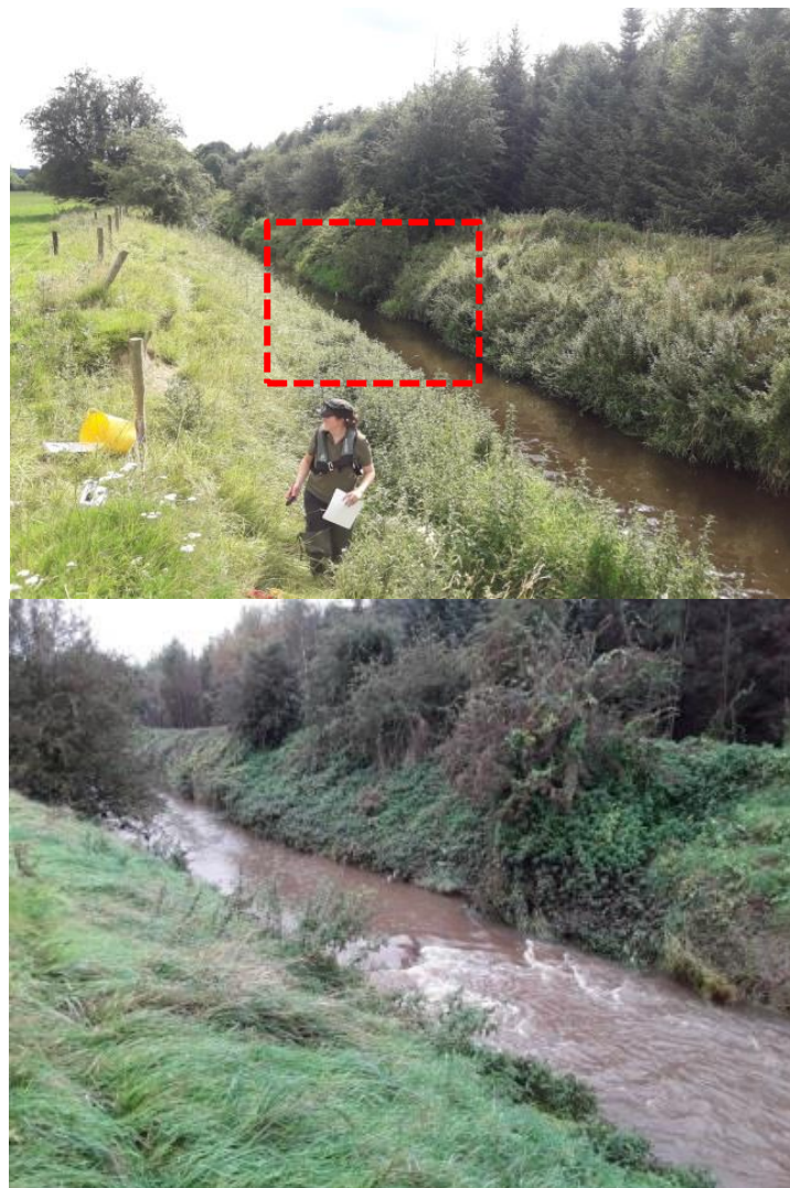
Figure 6.9 Example of pool excavation and riffle creation – before and after experimental digging.
