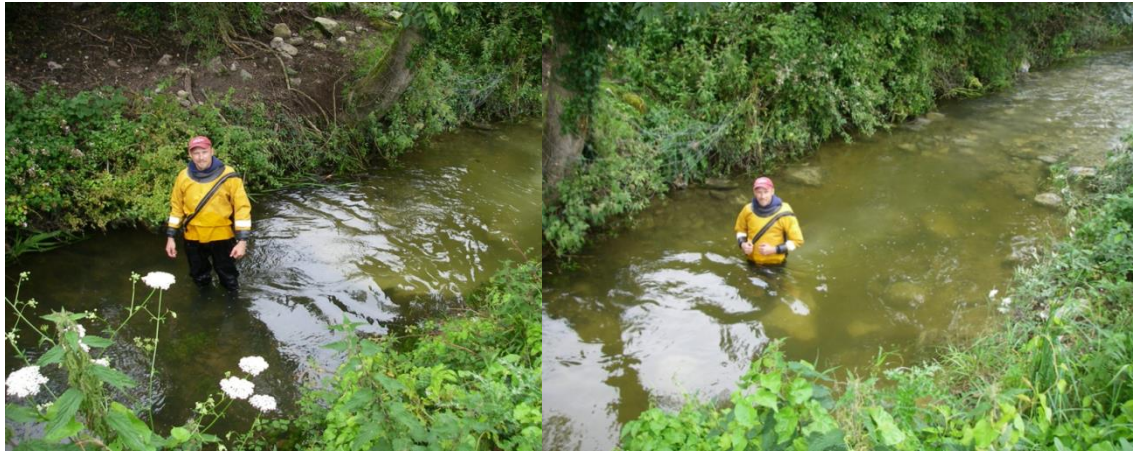
Figure 5.2 The Clonshire study site showing the pre-digging situation (left) and changes following bed excavation and formation of pool and riffle (right).
