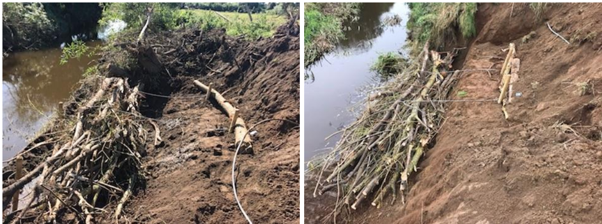
Figure 6.7 Soft engineering: willow bundles pinned to bank for reinforcement, which were then covered with a clay sod to incorporate the structure back into the bank.
