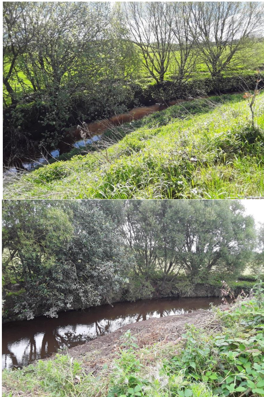
Figure 6.8 Example of berm management with retention of mature tree cover on the non-working bank.
