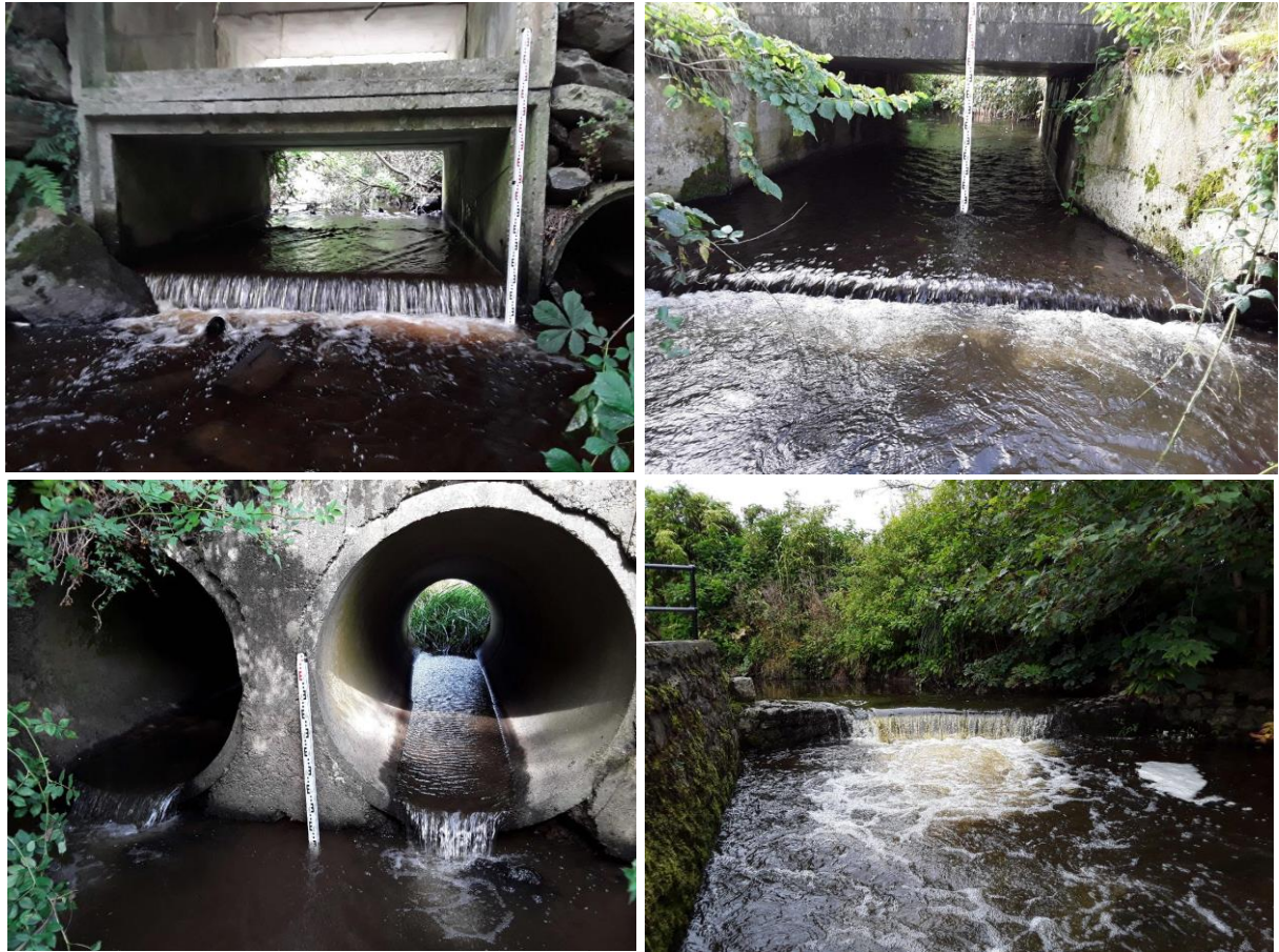
Figure 2.19 Examples of barriers identified during the Deel survey, including a box culvert, bridge apron, pipe culvert and small weir.
