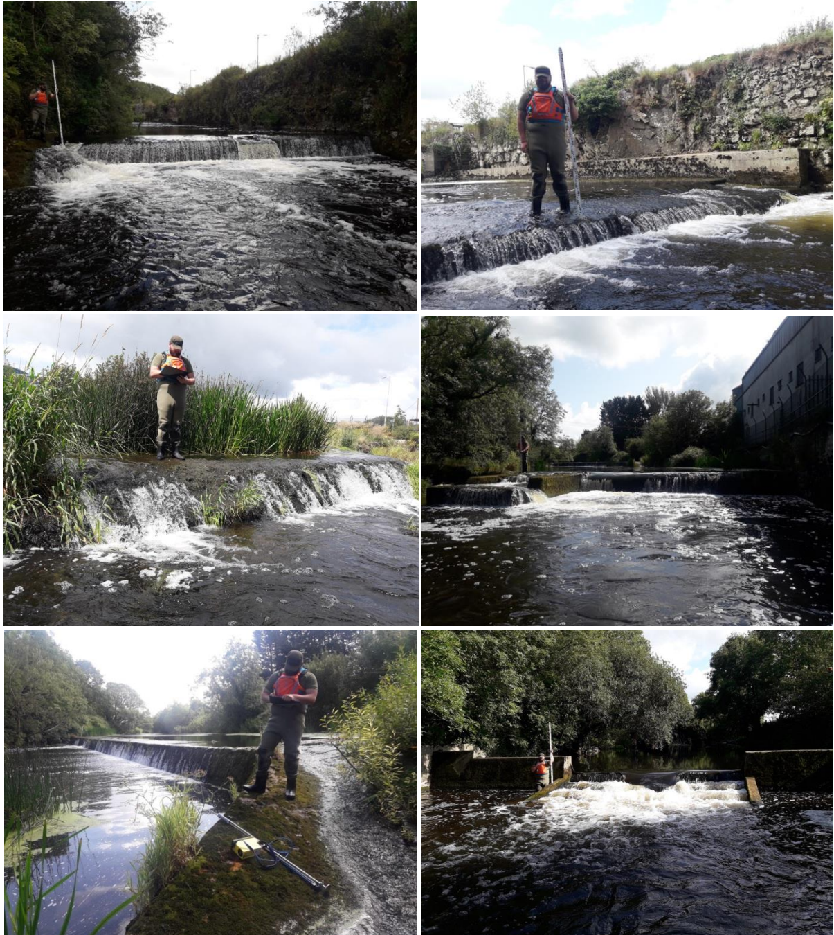
Figure 2.21 Askeaton weirs presenting barriers to migrating fish. Top row (1-2); middle (3-4); bottom (5-6).
