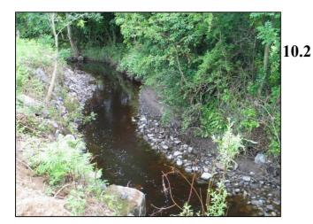
2 Overdeepen the channel along one side and place spoil on opposite side –particularly on curves and bends
