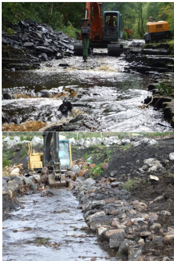
Figure 3. An example of the rehabilitation work carried out on the Owengar River
