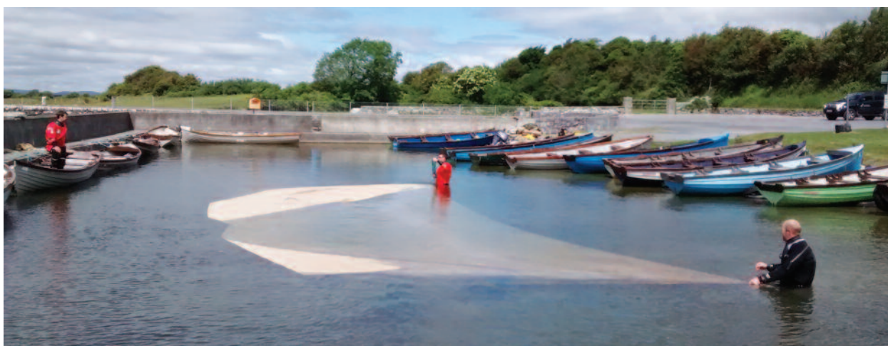
Laying a light excluding bio-degradable jute matting at two harbours in June
