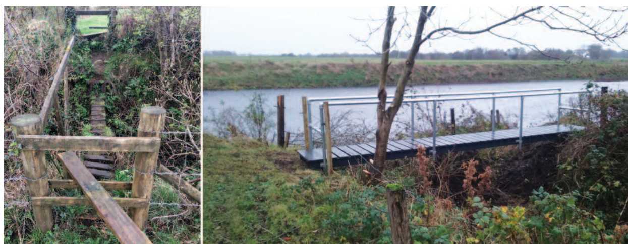
Dangerous bridge on the EMMA section of the River Moy (left) and one of the new replacement bridges installed in 2015 (right)
