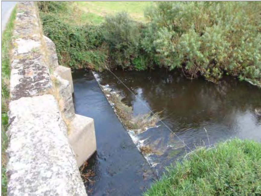
Plate 2.9 Barrier to lamprey passage on the Kells Blackwater at Stramaquerty Bridge, Virginia, Co. Cavan.
