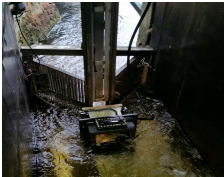
Plate 1 Erriff upstream adult fish trap with VAKI Riverwatcher counter and Biomark antenna (dark rectangular unit). Fish migrating upstream past Aasleagh Falls (tidal limit) enter through the trap door and are manually identified as sea trout or salmon (grilse or multi-sea winter); and ranched salmon are intercepted and removed. Detections of PIT tagged fish are registered and typically tagged fish are sampled for length, weight and scale sampled and released (see Section 4.2.1).
