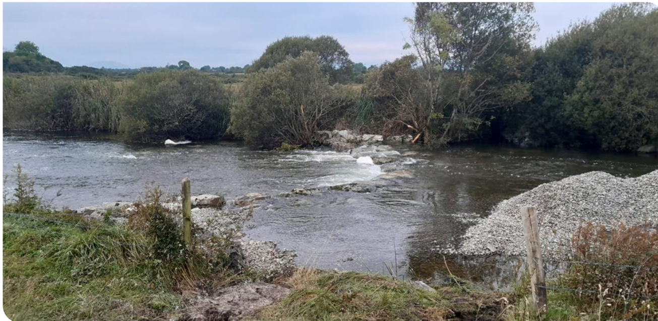
Image: Stone weir reshaped into upstream facing arc with spawning gravel to be redistributed up stream.
