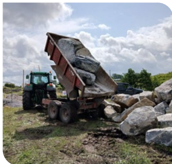
Image: Delivery of rock for building deflectors on the Togher River.
