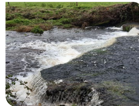
Image: Concrete Bridge Apron at Templederry, County Tipperary, pre-works photograph.
