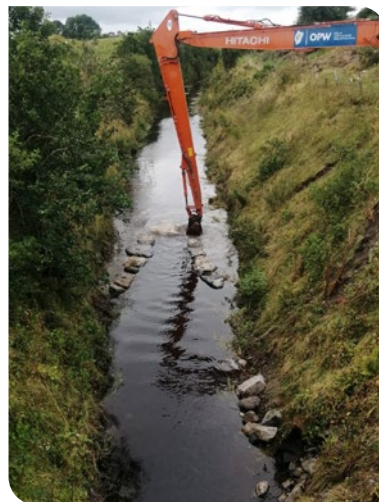
Image: Restoration of the Togher River site included introducing in-stream features such as deflectors.
