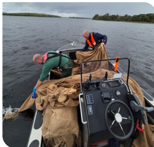
Image: Divers deploy jute matting from boats.
