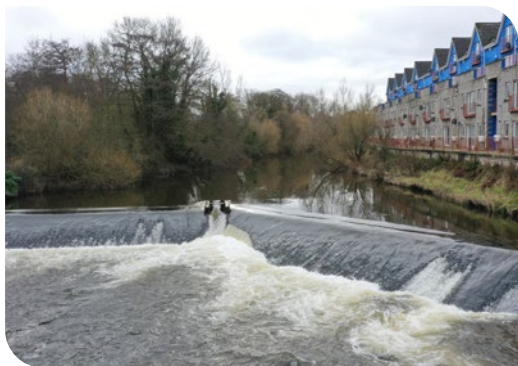
Image: Annacotty Weir - Barrier Mitigation project. Photograph of existing weir.
