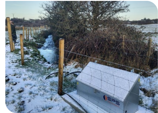
Image: Stock proof fencing erected and solar powered pumps installed.
