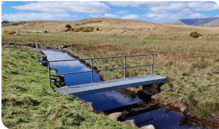
Image: Angler access bridge installed at Beat 2, Erriff Fishery.
