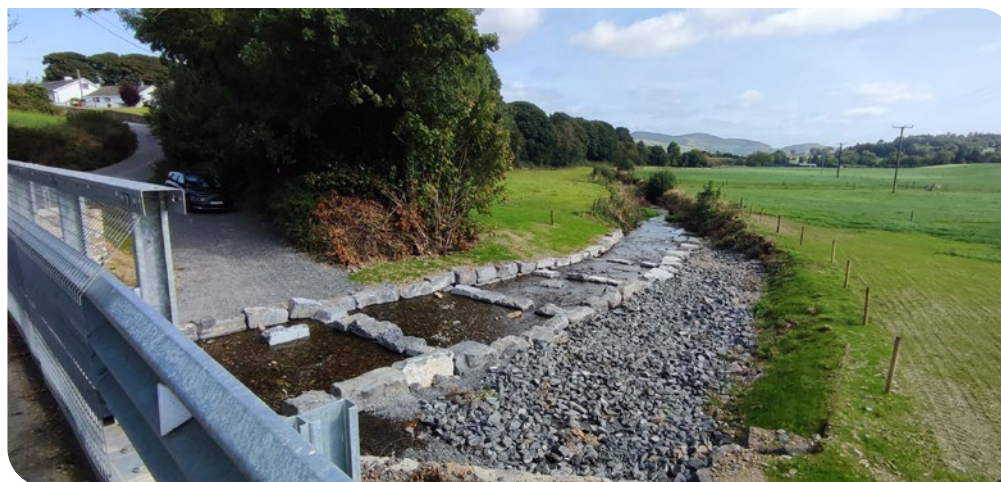
Image: Bridge at Templederry, County Tipperary, post-works photograph of new rock ramp fish pass.
