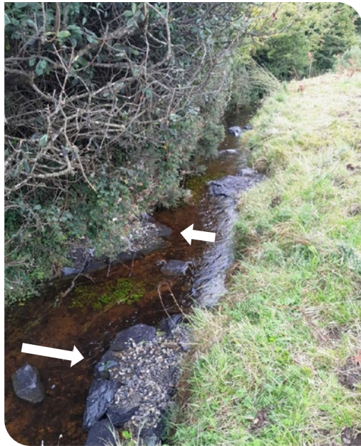
Image: Alternating deflectors and placement of random boulders in the Newtown River.
