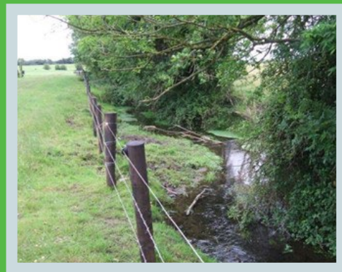
^ Yellow River Phase 2 fencing work 1
