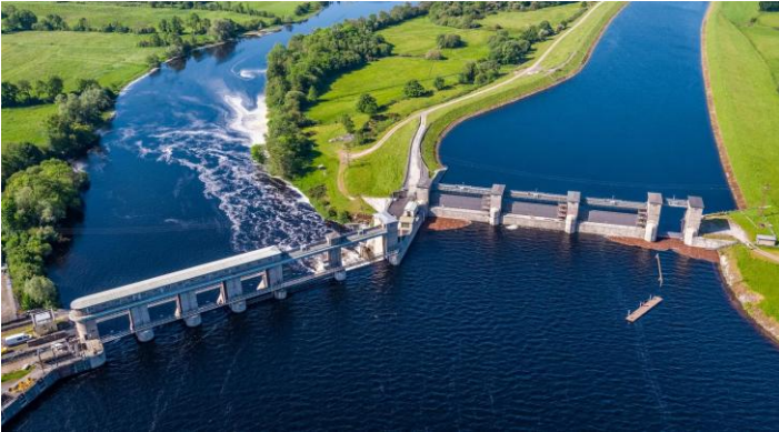
Plate 5-2 Aerial photo of Parteen regulating weir with the Headrace canal on the right and old river channel on the left.
