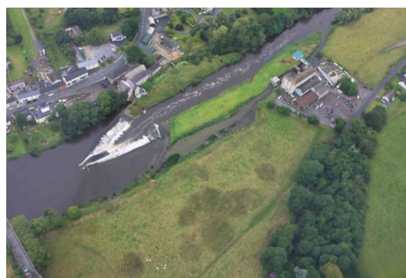
Figure 7 - Aerial photo example of mill tail and head race
