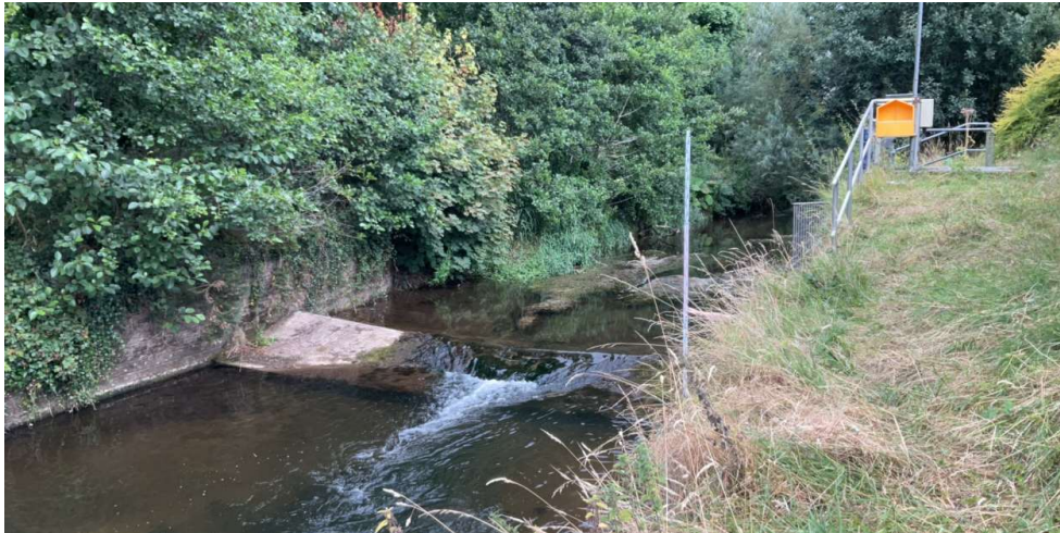
Figure 4.5 Weirs identified on the main stem of the Loobagh (C1/34). (Top: Sediment Trap [ST12]; Bottom: Gauging Station (24_729_24)).
