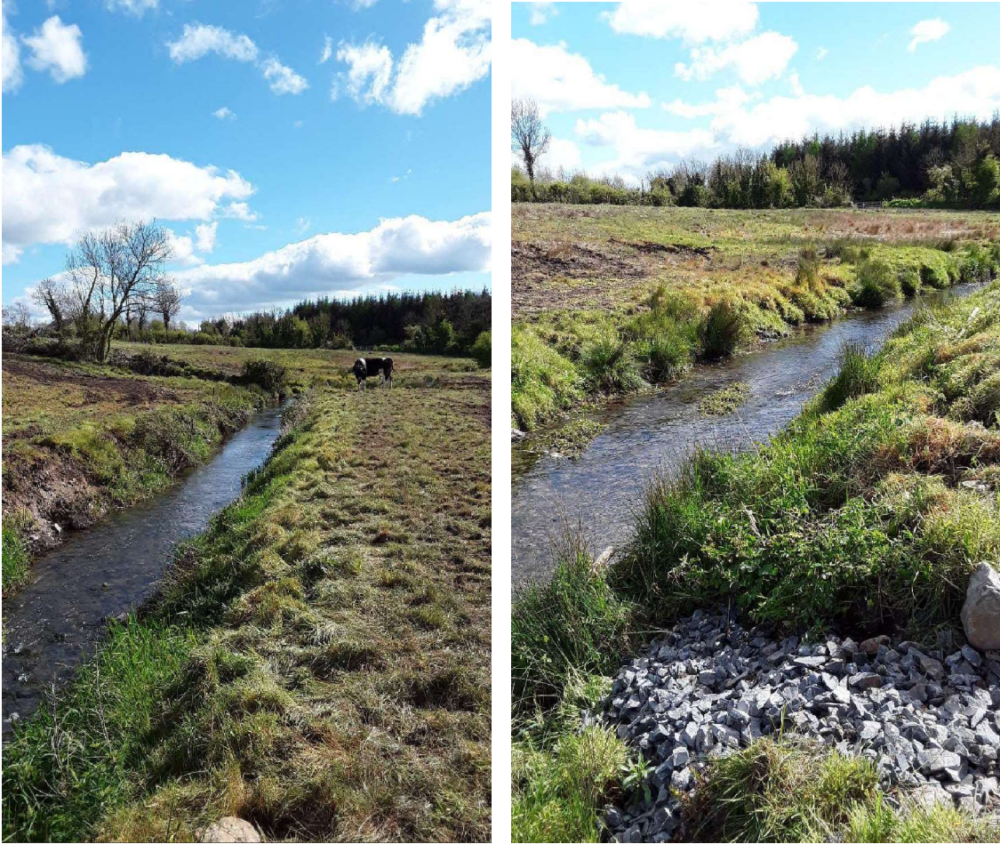
Figure 3.5 The Mahore River (C1/25/23) is heavily poached with unstable banks, large patches of closely cropped or bare ground and an absence of riparian cover. Vegetation is colonising the wetted area instream (right) demonstrating evidence the channel is over-widened.
