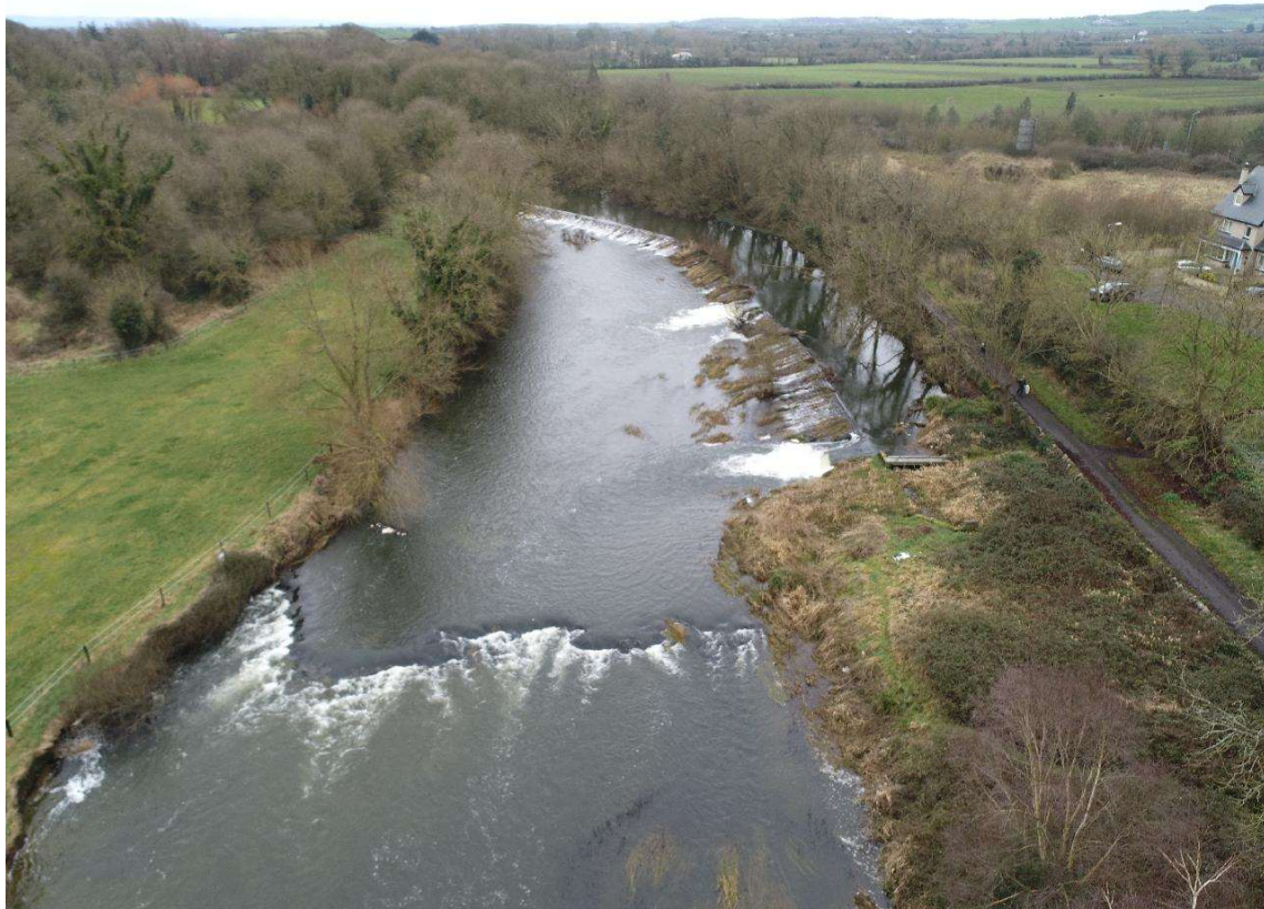
Figure 4.8 Drone imagery of the weir upstream of Croom. The weir has a crest width of 123 metres and a head height of 1.1 metres.
