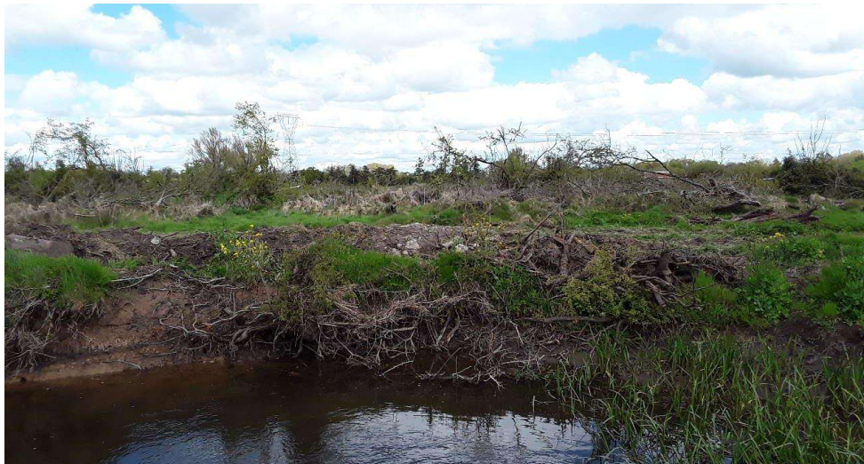
Figure 3.11 Poor land management where a small soil embankment was installed on the Drumcomoge River (C1/25) recently.
