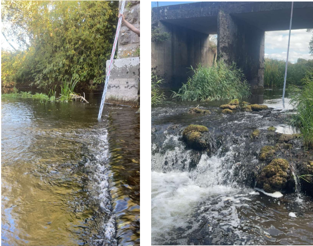
Figure 4.3 Problematic bridge aprons identified on the main stem of the Camoge (C1/25) (left: 24_711_42; right: 24_711_46).
