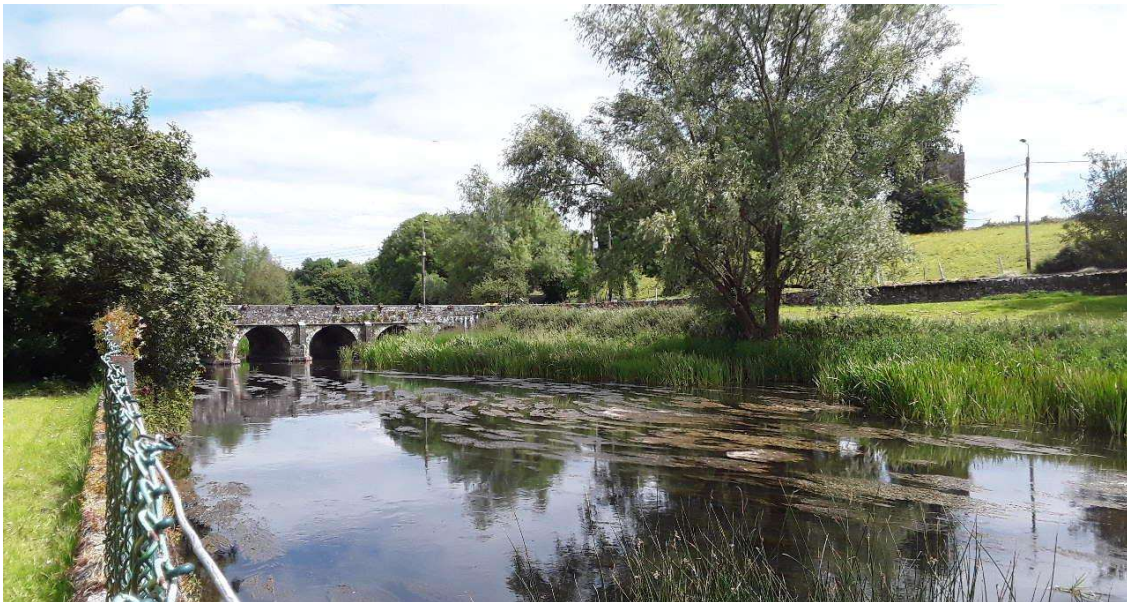
Figure 3.3 Impounded area upstream of the weir at Bruree (C1 Maigue Outfall).
