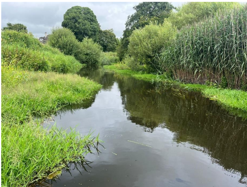
Figure 10. Lower Mount Nugent River vegetative growth encroaches on the channel.
