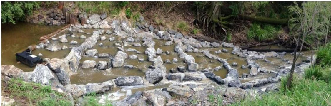
Figure 94. A full-width pool and boulder rock ramp fish pass designed to mitigate the impact of a weir on fish passage <https://catchmentsolutions.com.au/portfolio/rock-ramp-fishway/>.
