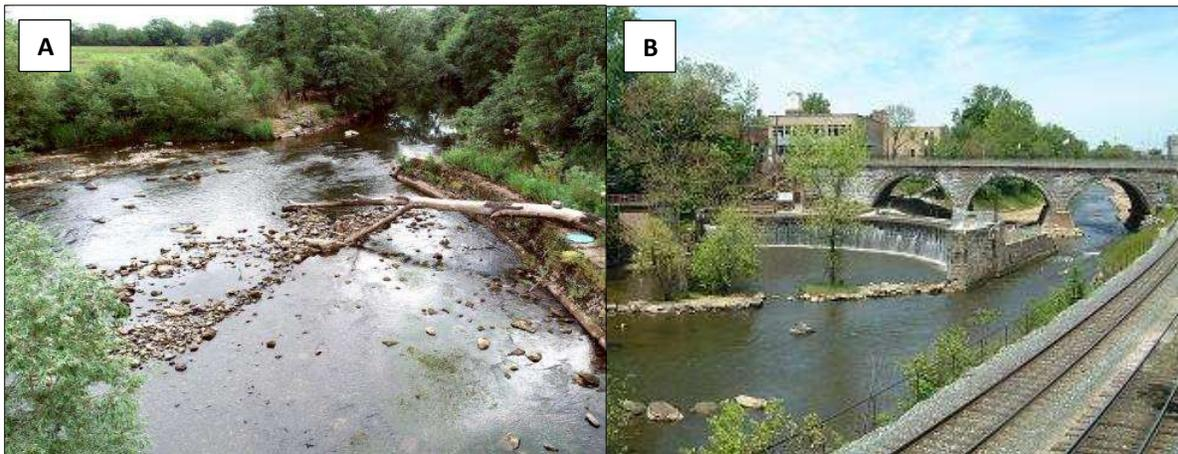
**Figure 89. Photos of breached weirs: (A) Ballyclough Weir in the Mulkear River, Co. Limerick, and (B) Kent Dam in the Cuyahoga River, Ohio, USA (breach in far right of image).**
