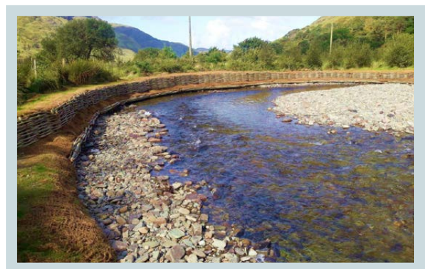
Willow weave bank revetment on the Glenamurra River Co. Mayo, carried out under the Salmon and Sea Trout Rehabilitation, Conservation and Protection fund, and completed in summer 2019.
