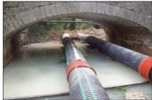
Repairs to a single arch bridge and scour slab with stream flow piped from upstream to downstream (foreground) during both grouting and slab repair.
