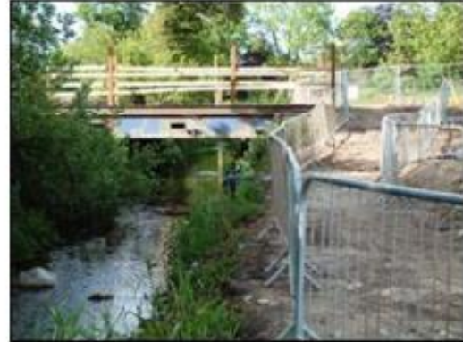
Temporary clear span 'Bailey bridge' ensuring free upstream and downstream movement of aquatic life. The streamside fencing should be 5 metres from the watercourse, not immediately alongside as in this photograph.
