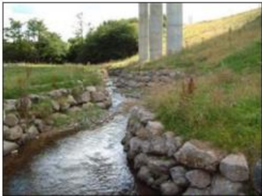
Suitably sized rock armour built to high water level at a location influenced by tidal back-up.
