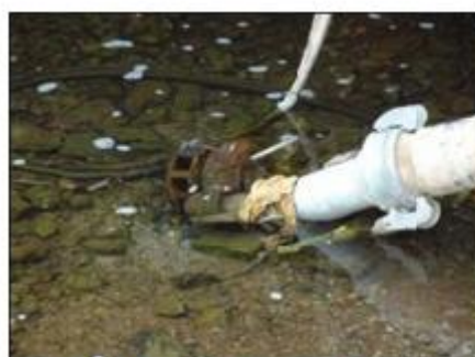
Continuous abstraction using submersible pump. No screening in place to prevent the entry of e.g. juvenile fish species to the pump. Unacceptable practice.
