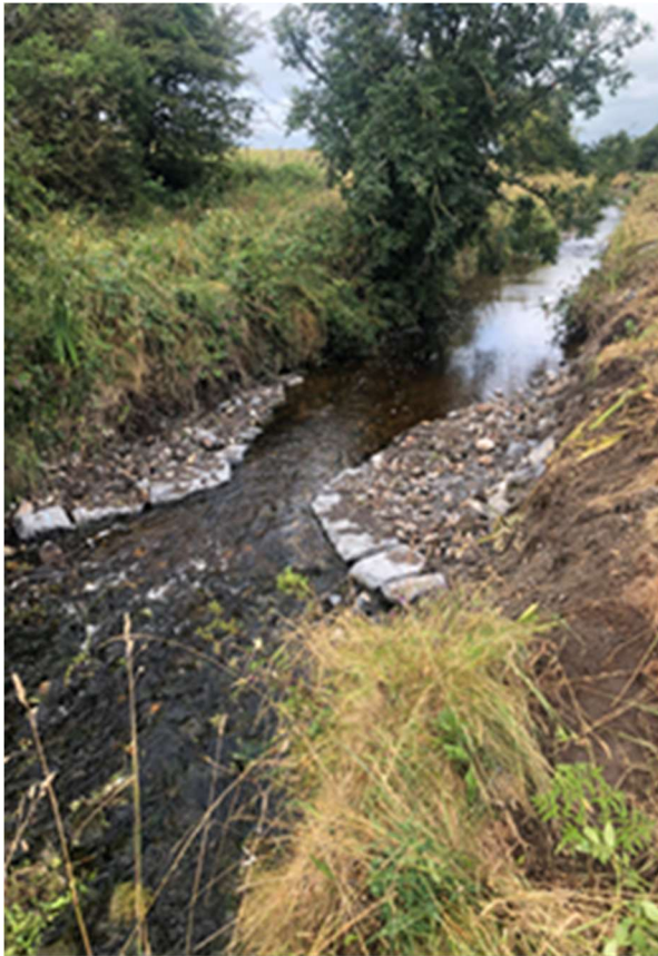
Fig. 9.1. Structures like the paired deflectors shown here help to vary flows and create more diverse hydrological conditions in arterially drained rivers. This helps to naturalise modified channels to improve biodiversity and conditions for salmonids. Fencing and strategic tree planting will also be carried out at many such sites to further enhance the recovery of watercourses to approximate their natural state
