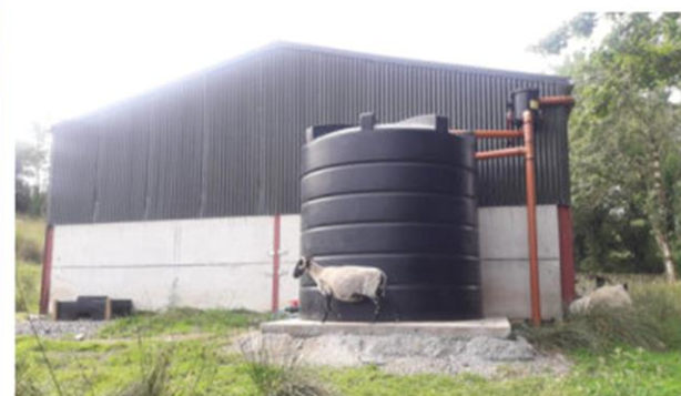
Rainwater harvesting installed at Blacklion Co Cavan
