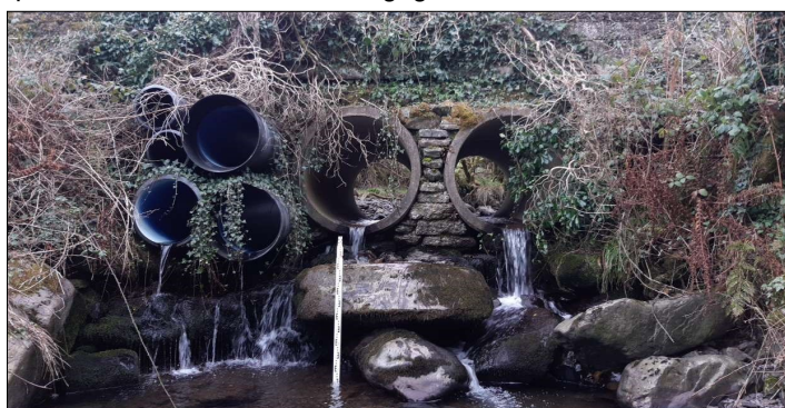
Road culverts are a common barrier to fish passage
