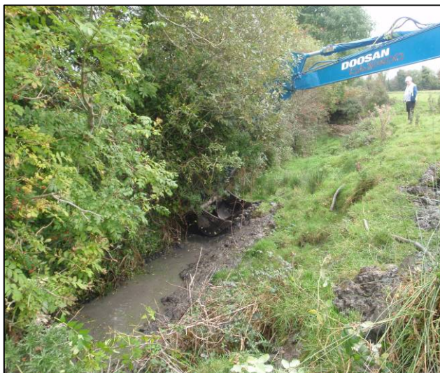
Plate 3.2. Machine bucket too big for channel it is working in.
