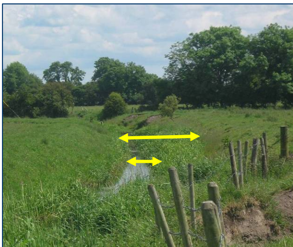
Plate 3.3. Design base width compared to desired base width.
