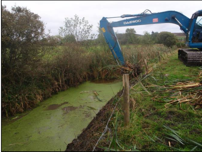
Plate 9.3. Excessive removal of instream and marginal vegetation and damage to non-working bank.
