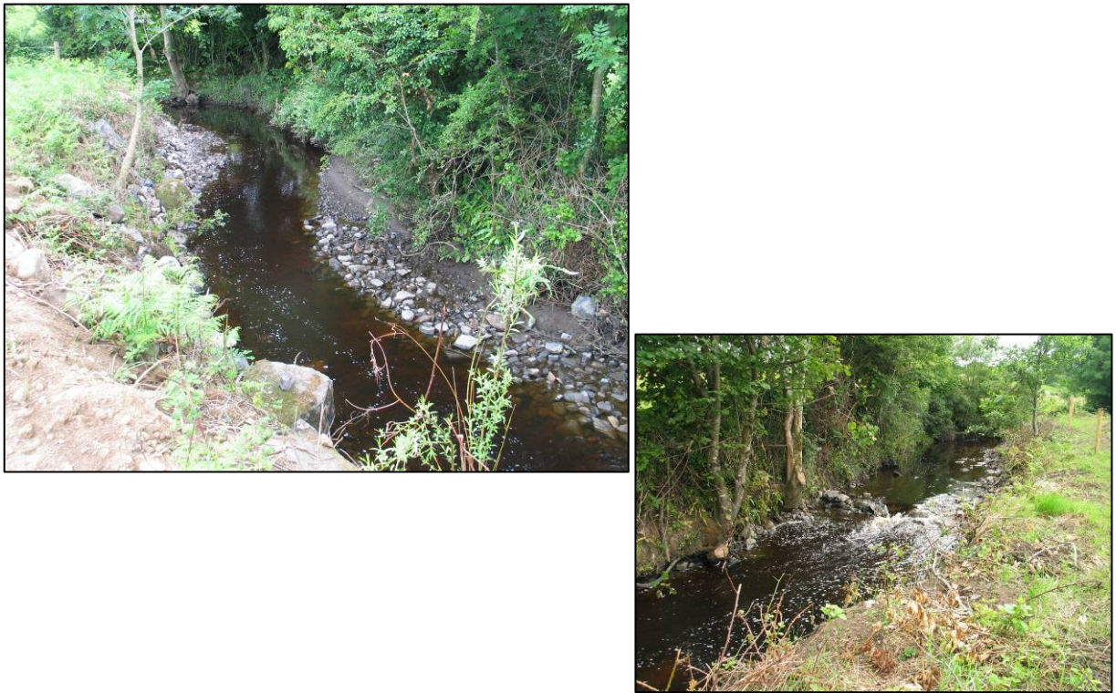
Plate 3.1. Examples of instream works carried out during Enhanced Maintenance on the Little R. Top left photo: series of alternating deflectors and digging out of a thalweg. Bottom right photo: creation of a weir and associated pool area downstream.
