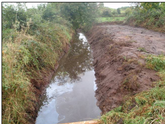
Plate 9.2. Excessive removal of bed material. Deposition of spoil on both bank slope and bank full line. Damage to non-working bank evident.
