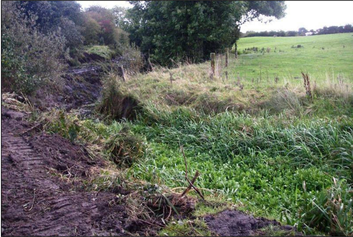
Plate 15. C40-2 (L. Ennel Tributary) Survey site during maintenance October 2008.
