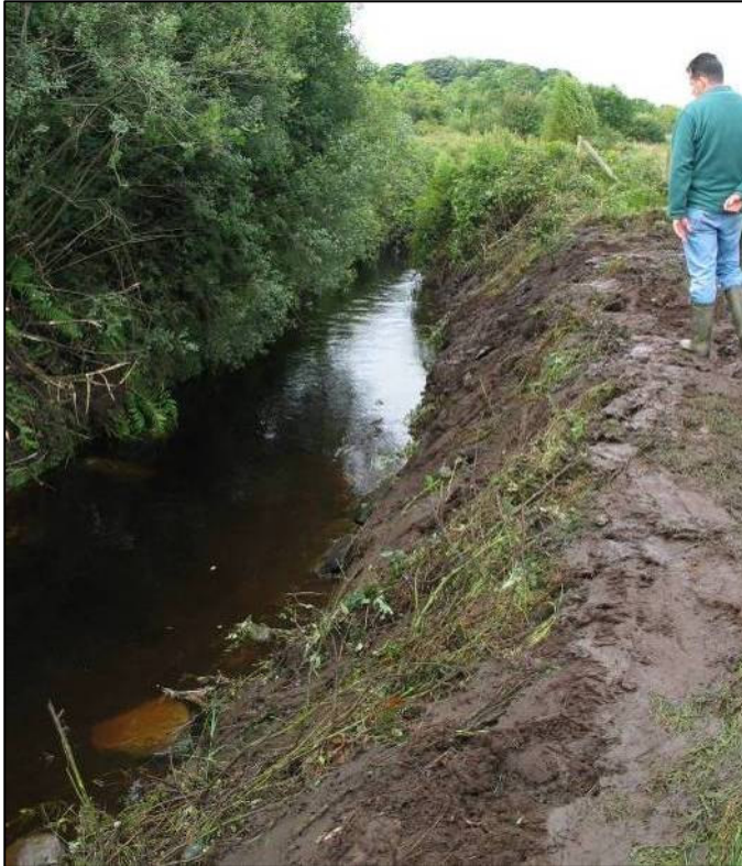
Plate 18. Excessive removal of all bank side vegetation from working side.
