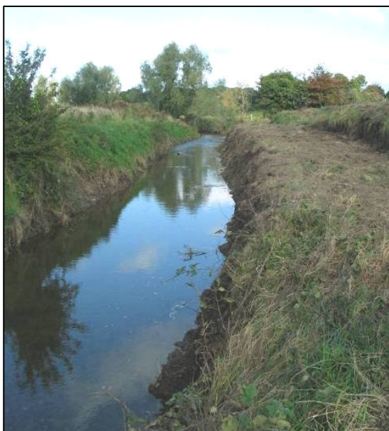
Plate 17. Both the bank slope and bank full cleared of vegetation
