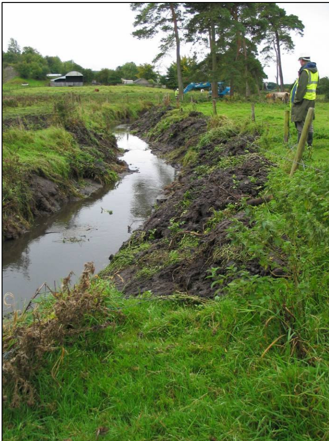
Plate 19. Excavated material deposited on the bank slope and damage also caused to the non working bank.
