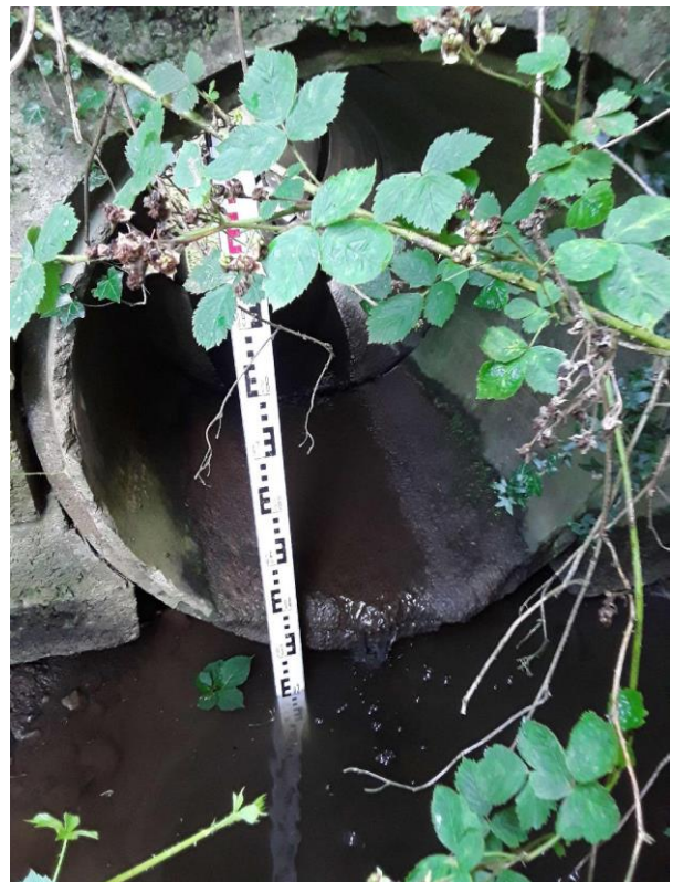
Figure 3.2 Examples of barriers on the Broadmeadow & Ward scheme. Bridge apron with drop, and perched culvert (top, C1/6). Two perched culverts (bottom, C2/10).
