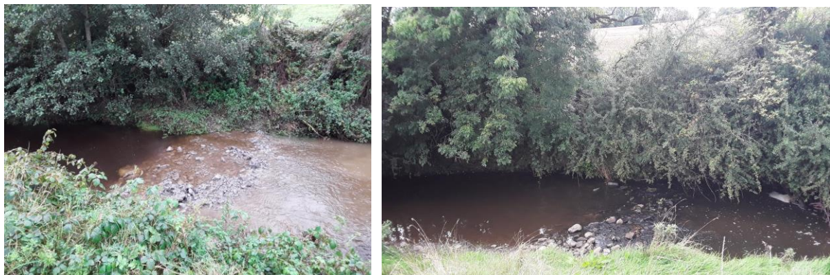
Figure 5.10 Left photo was taken post-works in 2019, and right photo was taken during a follow up walkover in 2021. It is evident that the pool and riffle remained intact.
