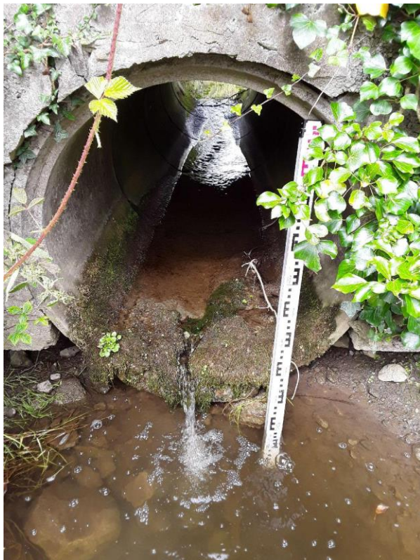
Figure 3.2 Examples of barriers on the Broadmeadow & Ward scheme. Bridge apron with drop, and perched culvert (top, C1/6). Two perched culverts (bottom, C2/10).
