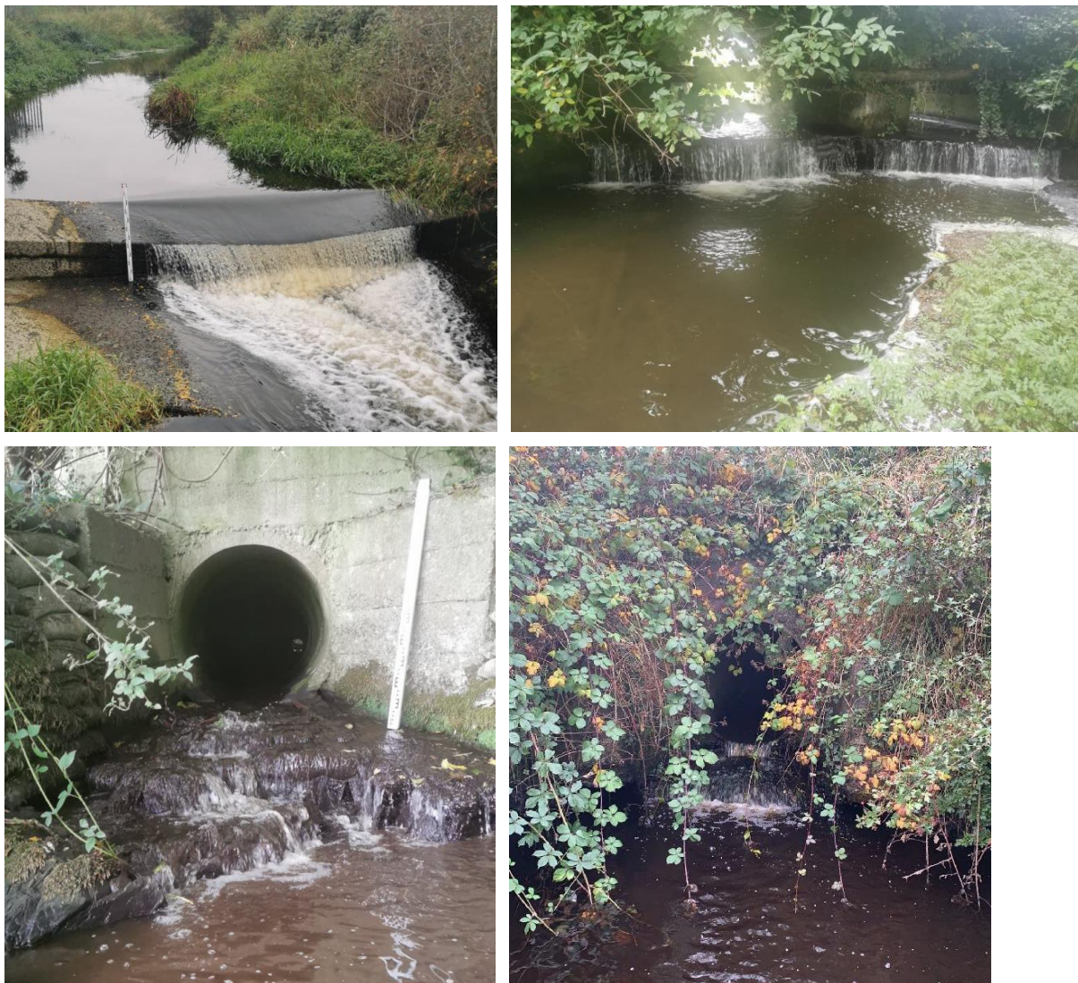
Figure 2.21 Small gauging weir (top left, C1/8/10); two-eye bridge with drop (top right, C1/8/15); culvert with apron and drop (bottom left, C1/8/16); perched culvert (bottom right, C1/8/19).
