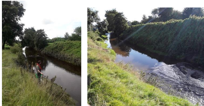
Figure 5.11 Left photo was taken pre-works showing a uniform glide and the photo on the right taken post-works. Changes in flows are evident following the introduction of paired deflectors which were created using the material from within the channel.
