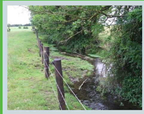
^ Yellow River Phase 2 fencing work 1
