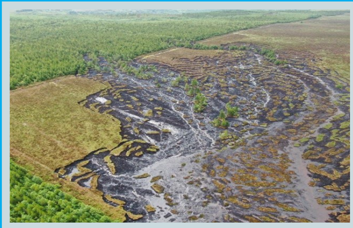
◀ The source of the Diffagher River Landslide, upstream of the Dawn of Hope Bridge, Co. Leitrim
