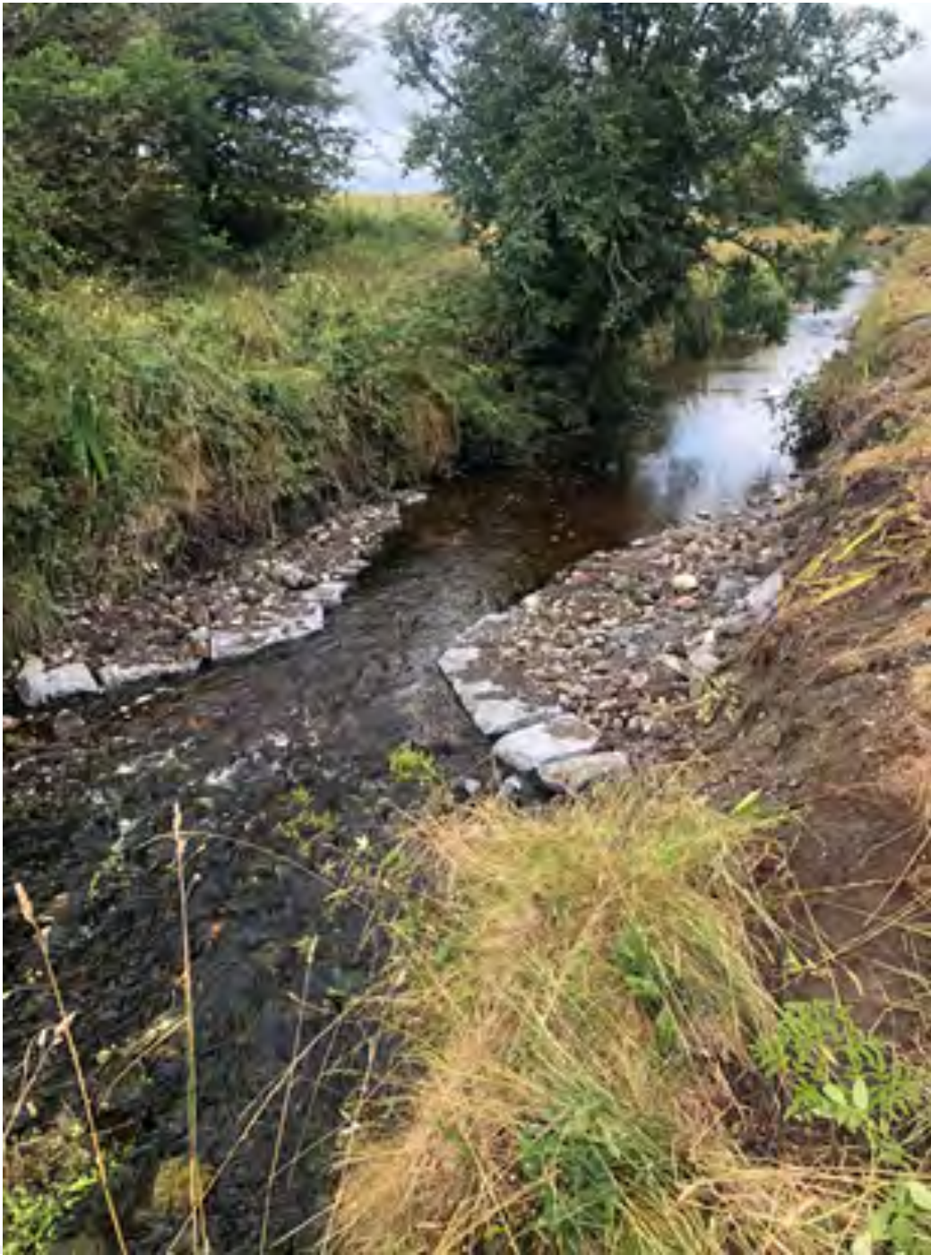
Fig. 9.1 Habitat Restoration: Structures, like these paired deflectors, help to vary flows and create more diverse hydrological conditions in arterially drained rivers. This naturalises heavily modified channels to improve biodiversity and conditions for
