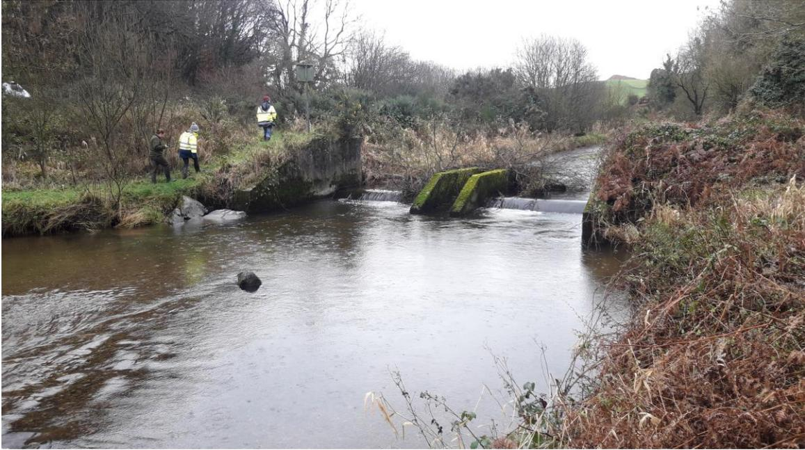
**Figure 4.1. Gravel trap on the main stem of the Nenagh River.**
