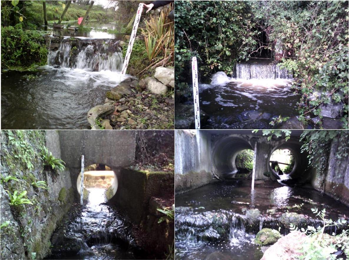
**Figure 1.15. Some of the barriers surveyed in the Northern Inny Basin during 2018 (standard levelling staff used for scaling).**
