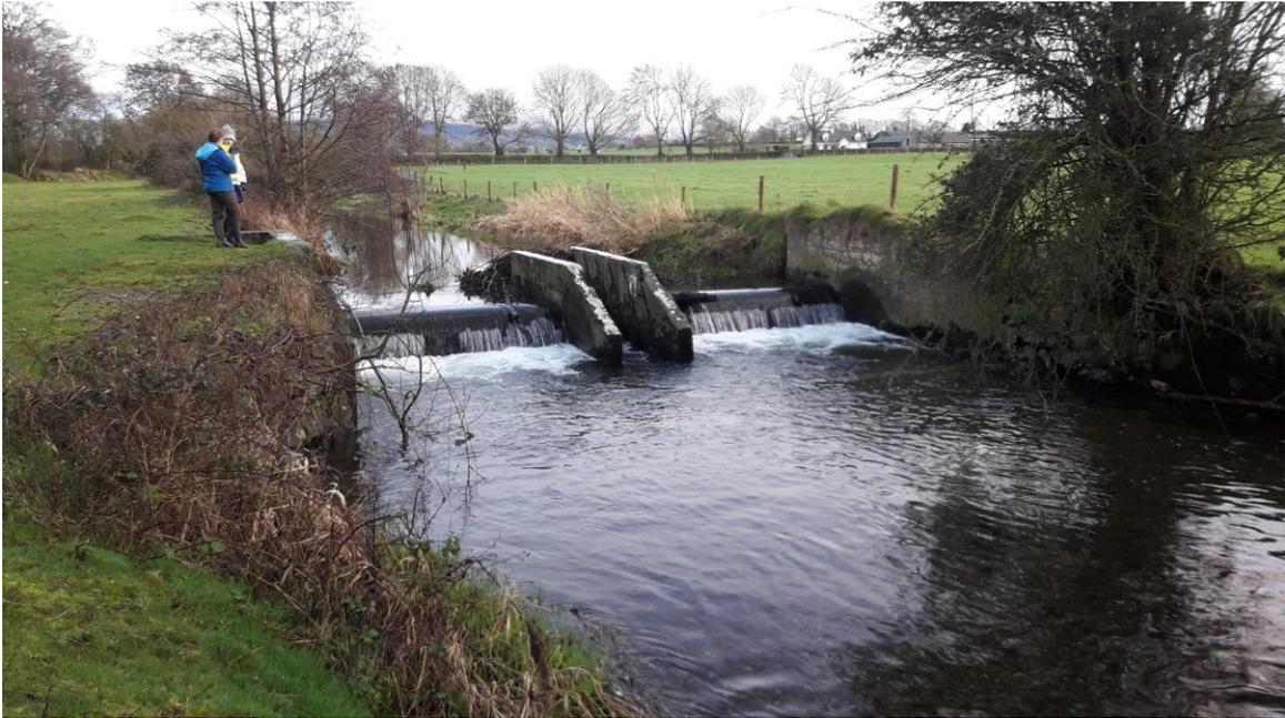
**Figure 4.2. Gravel trap on the Ollatrim River, in the Nenagh catchment.**
