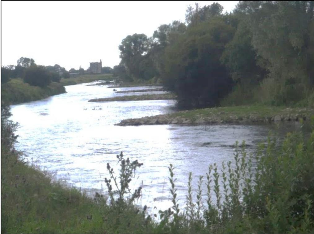
**Figure 2.5. Series of single deflectors around a bend, Boyne main channel (C1)**
