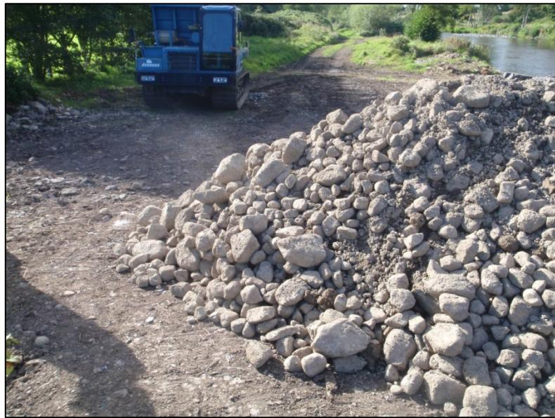
**Figure 2.2. Delivery of incorrect 'spawning gravels' (note the size range of the stone).**
