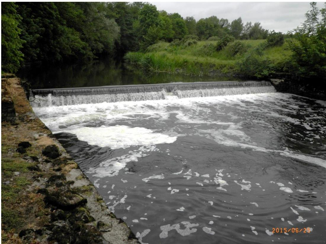
**Figure 5.4. Martry Mill on the Kells Blackwater (Boyne CDS) a structure highlighted for mitigation (rock ramp). This is a high impact barrier to adult salmon and a complete barrier to lamprey.**
