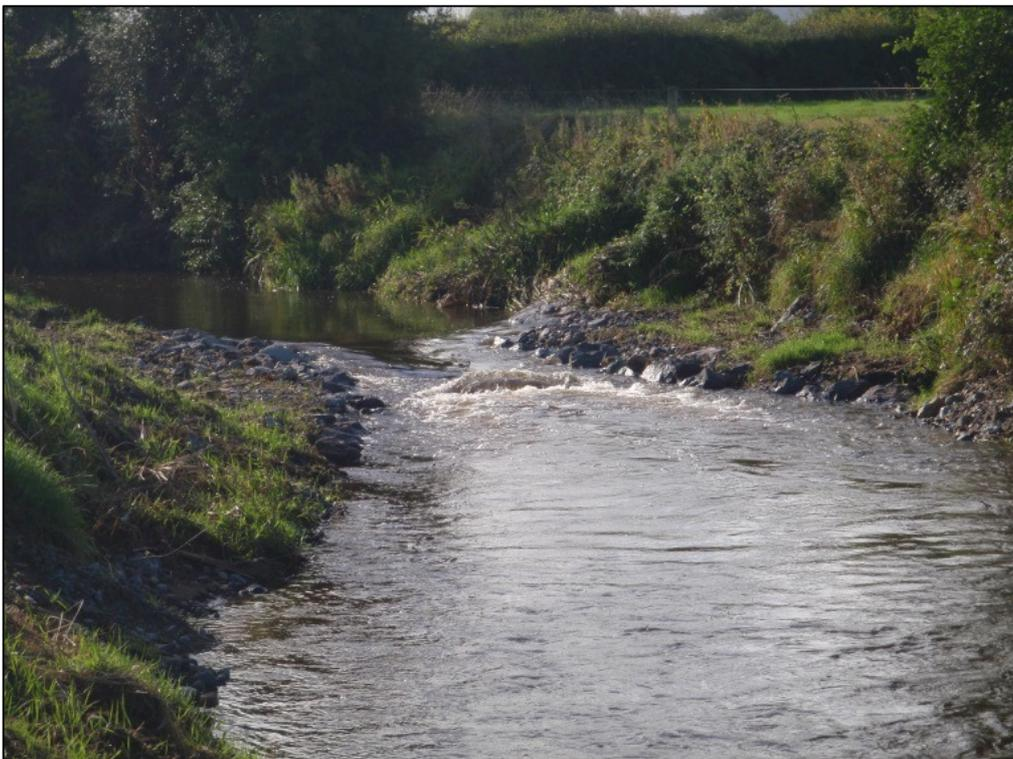
**Figure 2.6. Paired deflector, pool and gravel shoal unit, Loobagh River (Maigue C1/34)**
