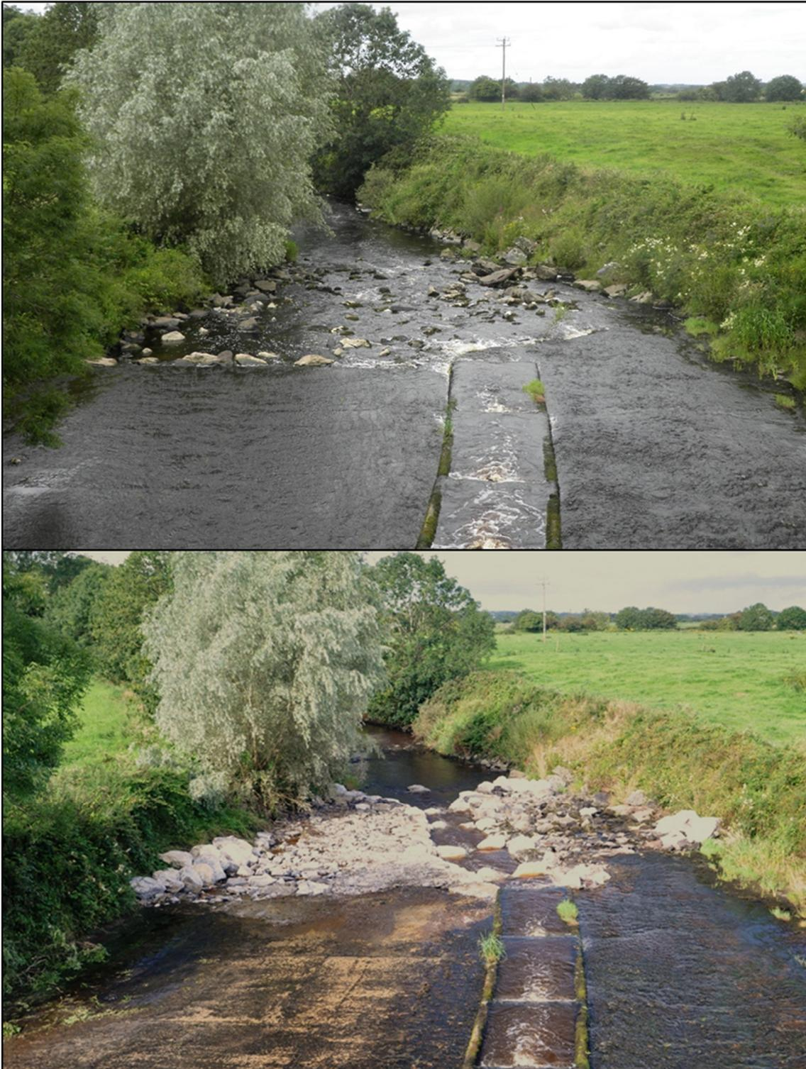
**Figure 5.3. 2015 remediation works at Ahavoher Bridge on the Galey River (Feale CDS), Pre (top) and Post (Bottom) works.**
