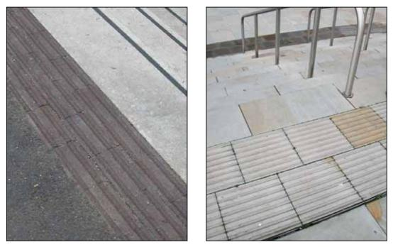
Hazard Warning units use continuous half-rods, raised 6mm higher than the surface of the paving, to denote a hazard, such as the top/bottom of a flight of steps. Again, the rods should be parallel to the edge of the hazard.
