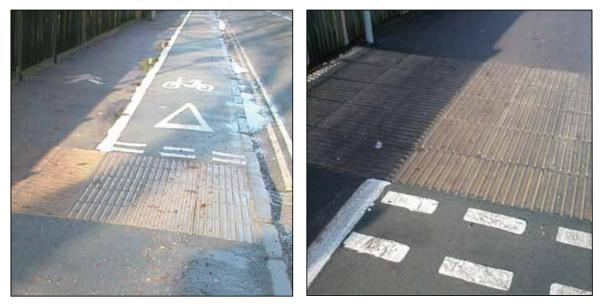
Where used to warn of an approaching flight of steps, corduroy paving should extend to the full width of the steps, plus at least 400mm to either side wherever possible. However, the corduroy paving must not extend across an adjacent ramp, access route or facility such as a lift.
