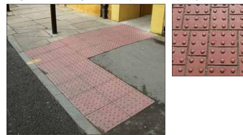
The Offset Blister units are used to indicate the edge of the platform at Rail and Tram stations, also referred to as off-street applications. Note that the orientation of the offset blister units is critical - the rows of blisters MUST be parallel to the platform edge, and they are generally placed approximately 500mm back from the edge. Image 1.38 Example of buff coloured offset blister units.
