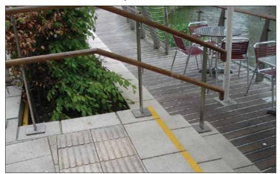
**Image 1.31** Example of exterior steps, corduroy hazard warning strips, top and bottom steps with contrasting colour strip, handrails plus landings. Note gap between handrails on each landing. The handrails should continue to help those needing additional support. Note also the lack of a permanent contrasting strip to the nosings of the steps between the top and bottom step plus there should be a tactile warning strip at the bottom of the steps.
