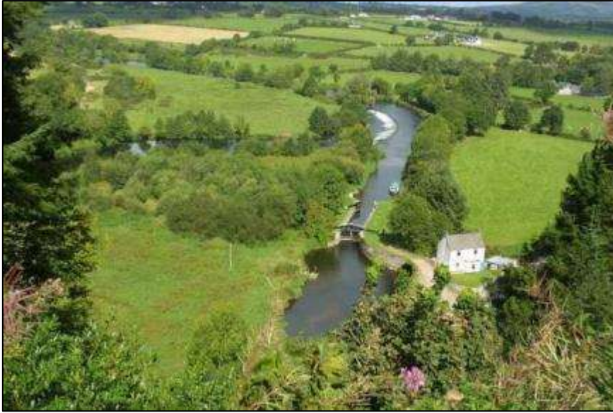
Plate 1.4. Example of a canal cut on the River Barrow at Clashganny, Co. Carlow.
