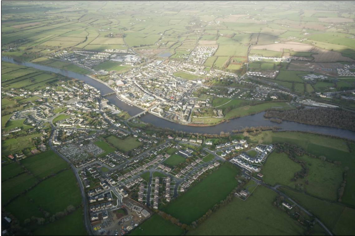
Plate 3.9. Aerial photo of the Upper Suir Estuary looking north over Carrick-on-Suir. (Photo courtesy of IFI and No. 3 Operational Wing, Irish Air Corps [Aer Chór na hÉireann])
