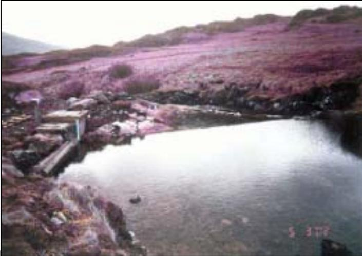
A high-head run of the river intake using a constructed river weir. Downstream view.
