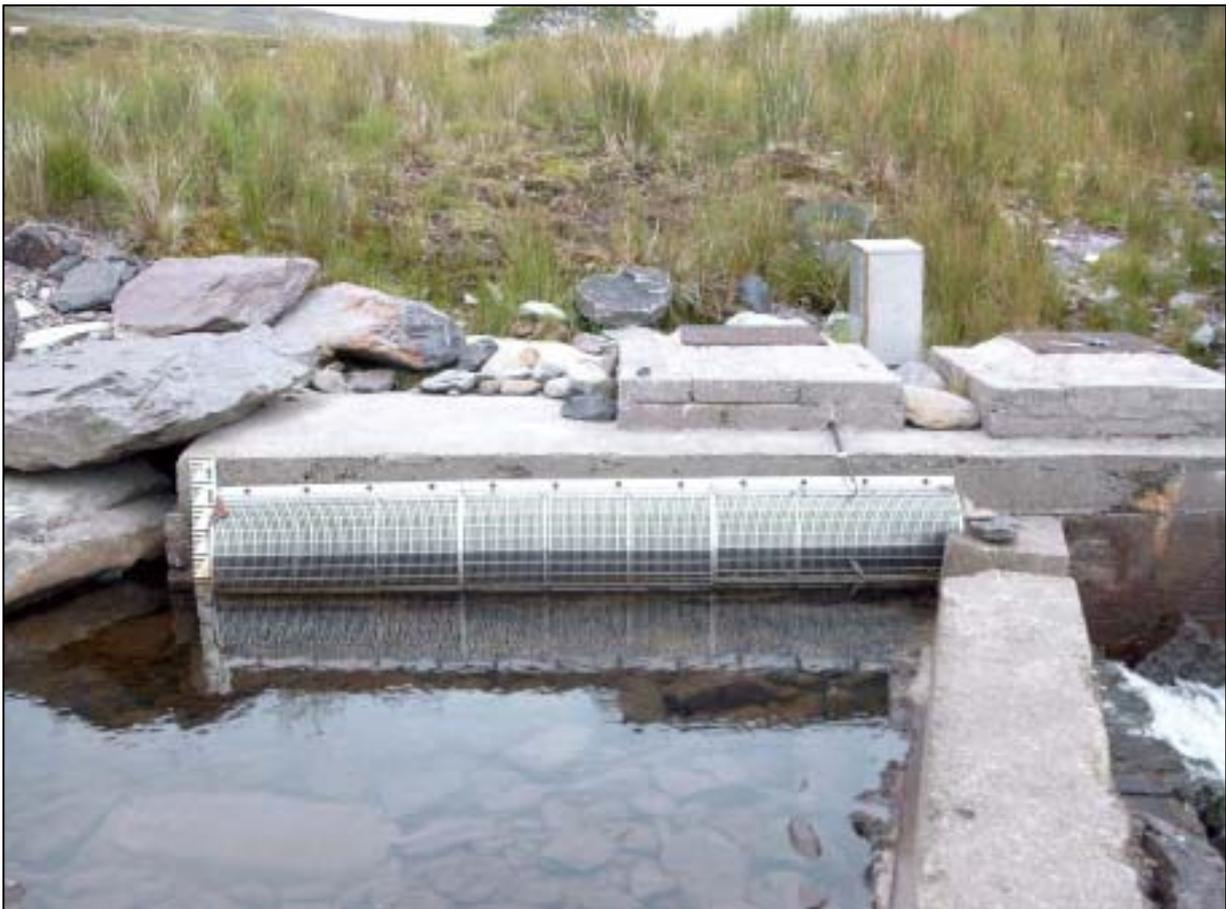
*Intake screen arrangement at a high-head site.*
