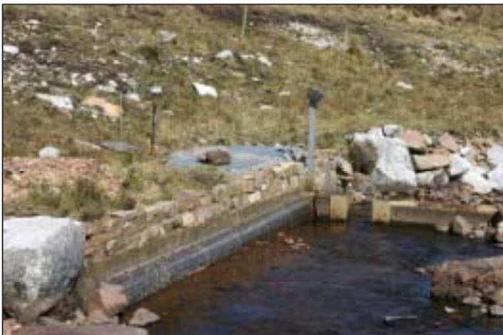
An example of the intake structure of a high-head run of the river using a constructed river weir. Downstream
