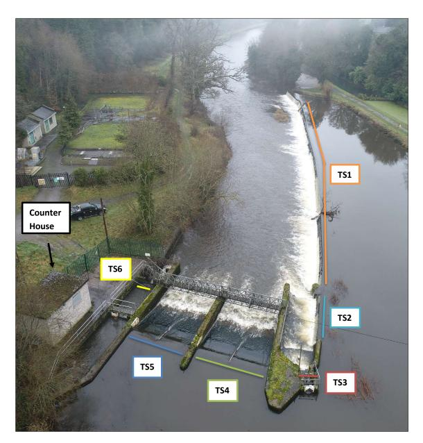
Figure 82. Blackcastle weir with transversal sections (TS) marked.
