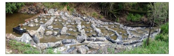
Figure 94. A full-width pool and boulder rock ramp fish pass designed to mitigate the impact of a weir on fish passage <u>https://catchmentsolutions.com.au/portfolio/rock-ramp-fishway/.</u>
