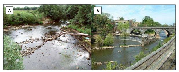
Figure 89. Photos of breached weirs: (A) Ballyclough Weir in the Mulkear River, Co. Limerick, and (B) Kent Dam in the Cuyahoga River, Ohio, USA (breach in far right of image).
