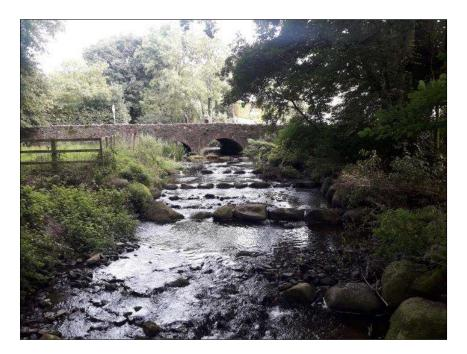
Figure 92. A full width pool and boulder rock ramp type fishway at Tuckmill Bridge, River Slaney, designed to mitigate the barrier impact of a bridge apron/culvert.
